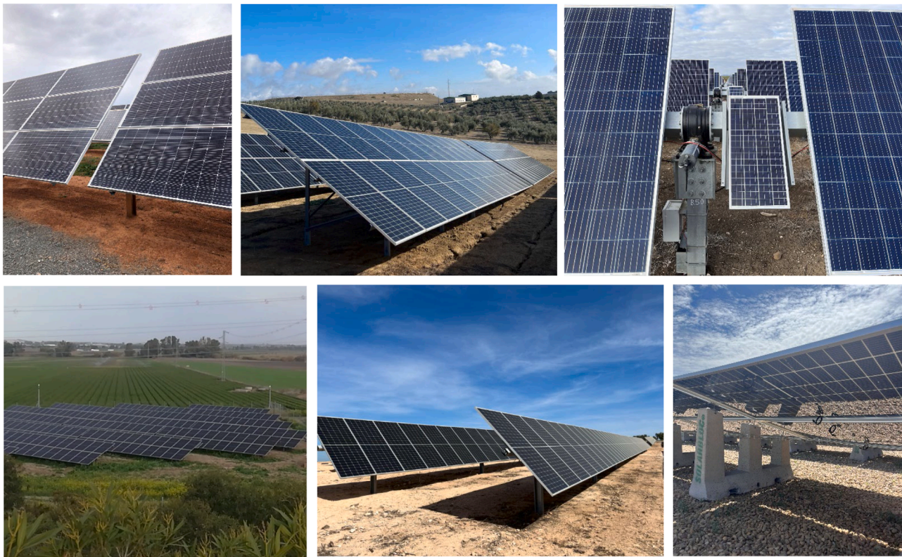
Fig. 2. Solar plants in the six irrigation systems. From top to bottom, left to right: solar panels with tracking system in the Valle Inferior system, where the small solar panel in between the panels is used for the tracking; fixed solar panels in the Santa María Magdalena system; solar panels with tracking system in the Bembézar system; fixed solar panels in the Guadalcaén system; solar panels with tracking system in the Genil Cabra system; and bifacial panels in the Zújar system.
