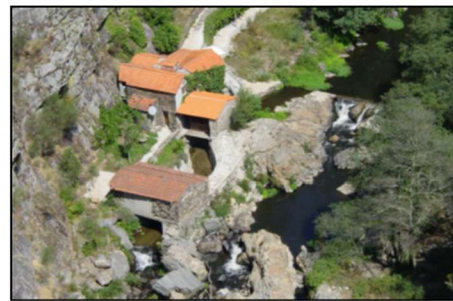
Figure 4. Existing stone weir at Moinho do Salto used to divert water into the historical mill channel.
