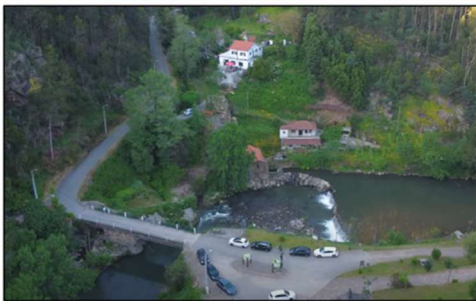
Figure 4. Existing stone weir at Moinho do Salto used to divert water into the historical mill channel.
