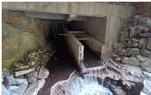
Figure 5. Partially preserved hydraulic channel leading water from the weir to the mill building.
